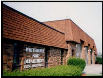
Whitehouse Fire Station
