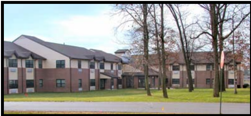
Spring Meadows Extended Care Facility Expansion
