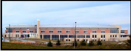
Miscellaneous Renovations at Bay Park Hospital
